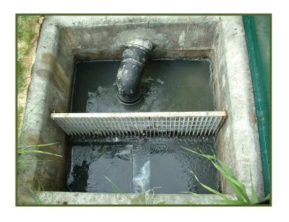
Basins are made by excavating the soil for a depth of about 1.2 m, are water-proofed by a geo-textile membrane in Pead, and are filled with design gravels.
