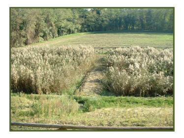
A device at the end of the basins allows to maintain the wastewater constantly under the surface of the bed, avoiding aerosols, bad odours and insects development, being the plant near to houses. In the basins have been planted native vegetal species (*Phragmites Australis*).
