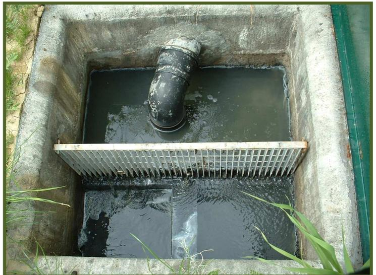
Basins are made by excavating the soil for a depth of about 1.2 m, are water-proofed by a geo-textile membrane in Pead, and are filled with design gravels.
